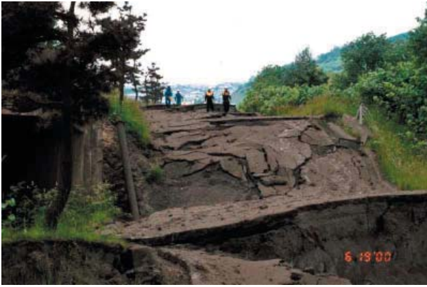
The road drastically changed in shape due the crustal deformation
