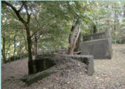
Uplifted Bridge Remain Park
